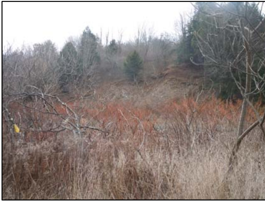
View of failure 6 from opposite side of brook
