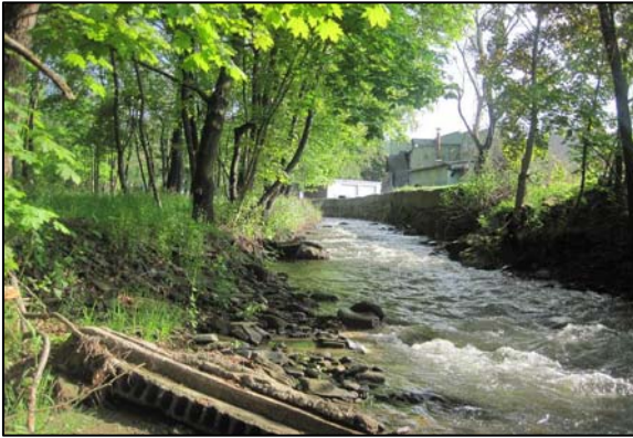
Rock wall bank revetment behind Klinger facility and Jake's Garden Supply
