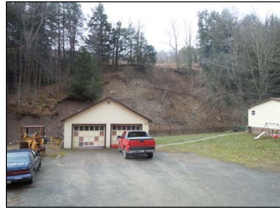
View of failure 9 from opposite side of brook
