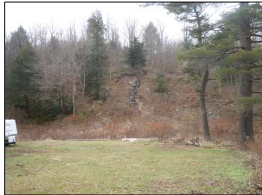
View of failure 5 from opposite side of brook
