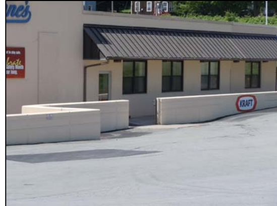
Existing Low Wall at Kraft Facility
