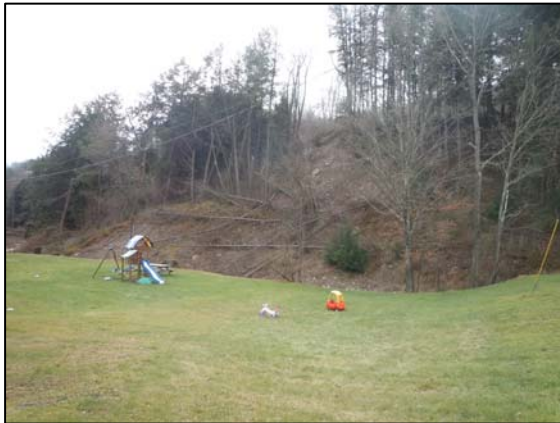
View of failure 8 from opposite side of brook
