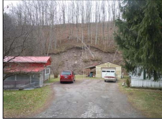
View of failure 3 from opposite side of brook
