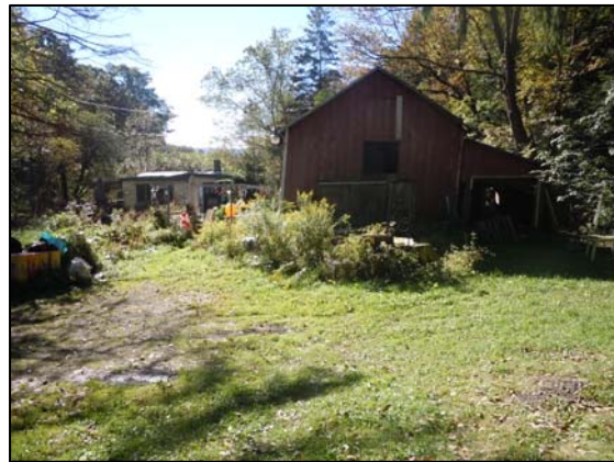
Barn at 757 Lower Third Brook Road is one of the few structures in the FEMA SFHA.
