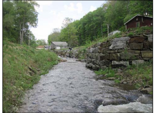
Third Brook main stem near station 72+50, facing upstream
