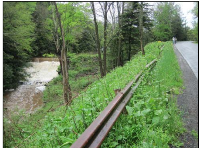
Old Village Reservoir dam
