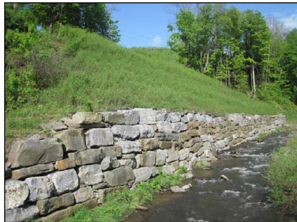
Stacked rock wall bank revetment near station 36+00
