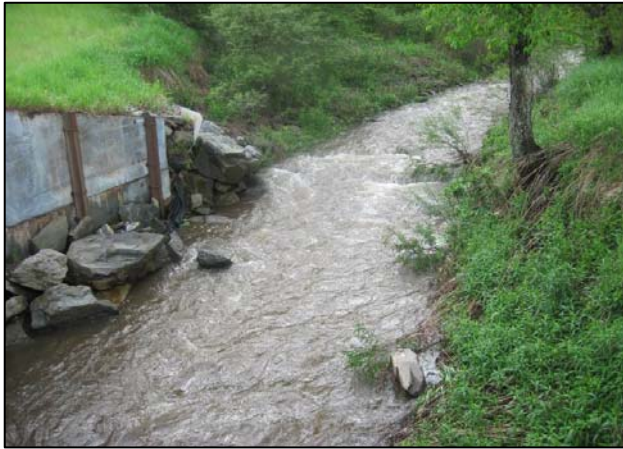
Third Brook main stem approaching Lower Third Brook Road bridge
