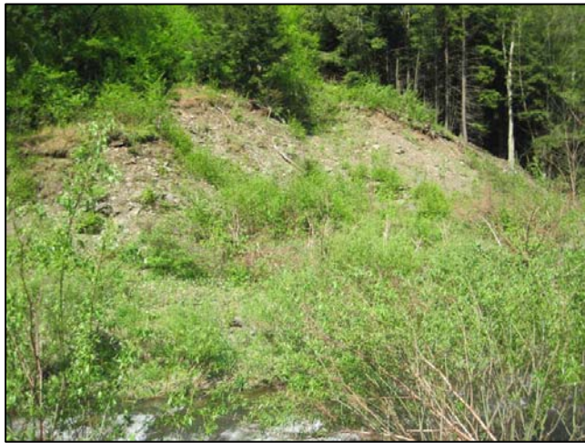
Bank slope failure near station 58+00
