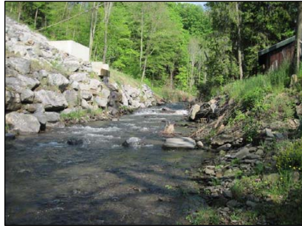
Incised channel with riprap slope stabilization on the right descending bank
