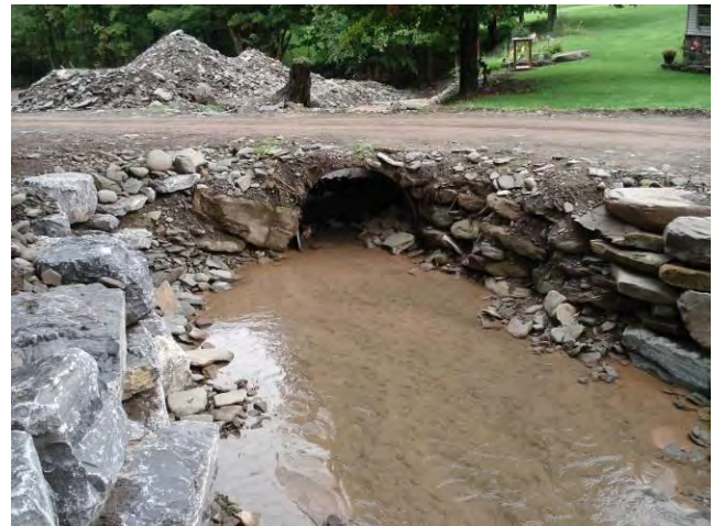
Figure 2.17 Culvert Conveying Holliday Brook Colchester, NY
