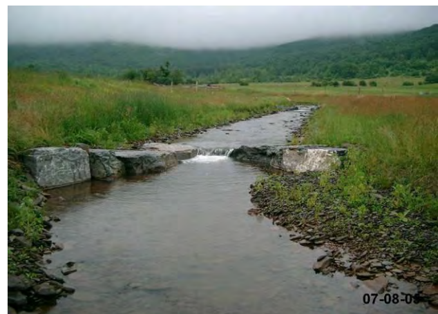
Figure 3.17 Rock Cross-Vane
