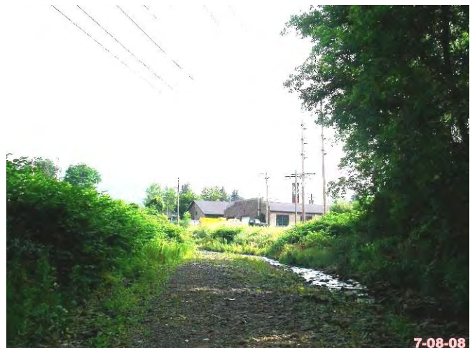
Figure 3.14 Two years later after Post Flood Intervention.
