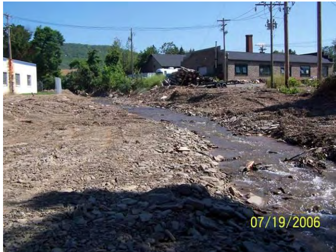
Figure 3.13 Shows stream channel after Post Flood Intervention.
