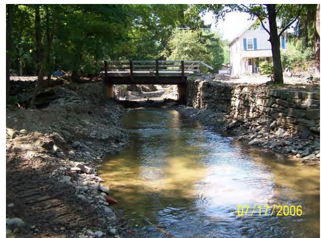
Figure 2.18 Bridge with no floodplain
