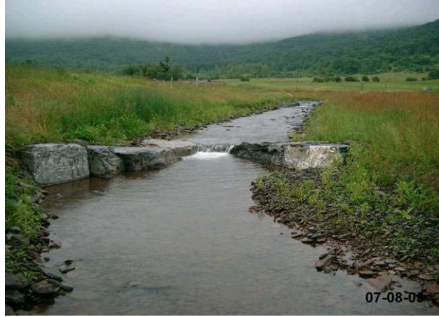
Figure 3.19 Rock Cross-Vane
