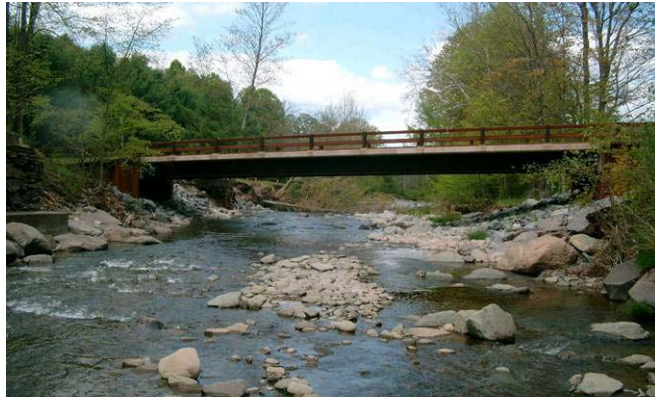
Figure 3.14 Bridge at Erpf Road
