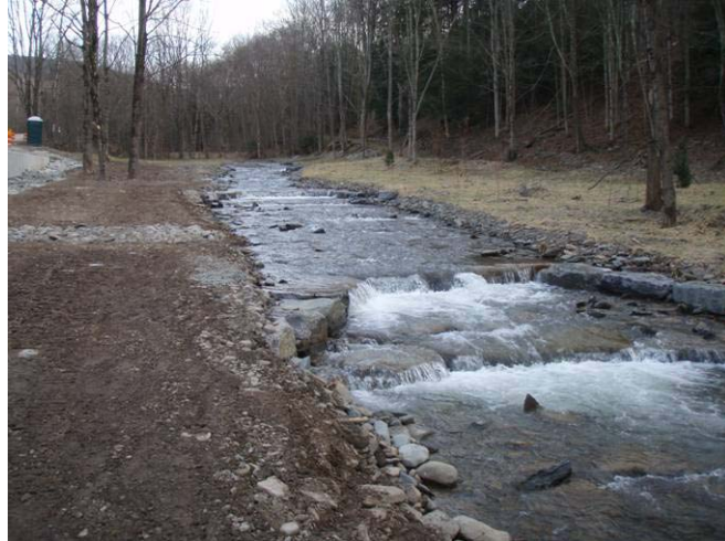
Figure 9.3 Holliday Brook After Construction with Cross Vane Structure
