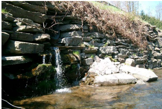
Figure 3.13 Dry Brook Road Culvert
