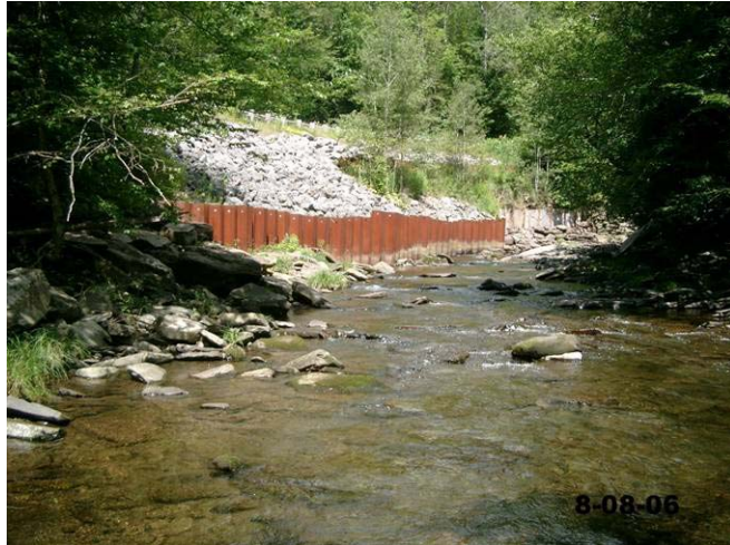
Figure 1.9 Revetment for Road Protection
