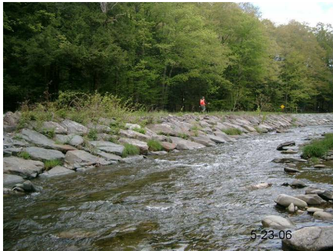
Figure 1.6 Rock Revetment Along Ulster County Route 49
