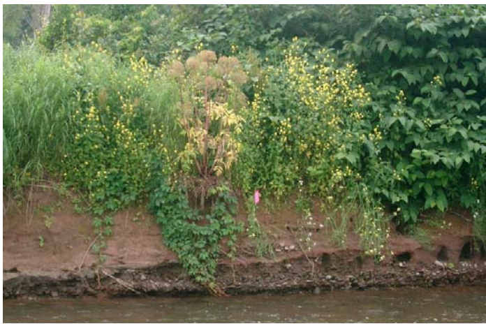
Figure 7.4.10 Poorly vegetated bank and a section of Japanese knotweed located approximately 2,000 feet upstream from County Bridge 10.
