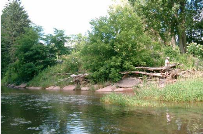
Figure 7.4.8 Rip rap along the island upstream from Kingston Street Bridge.
