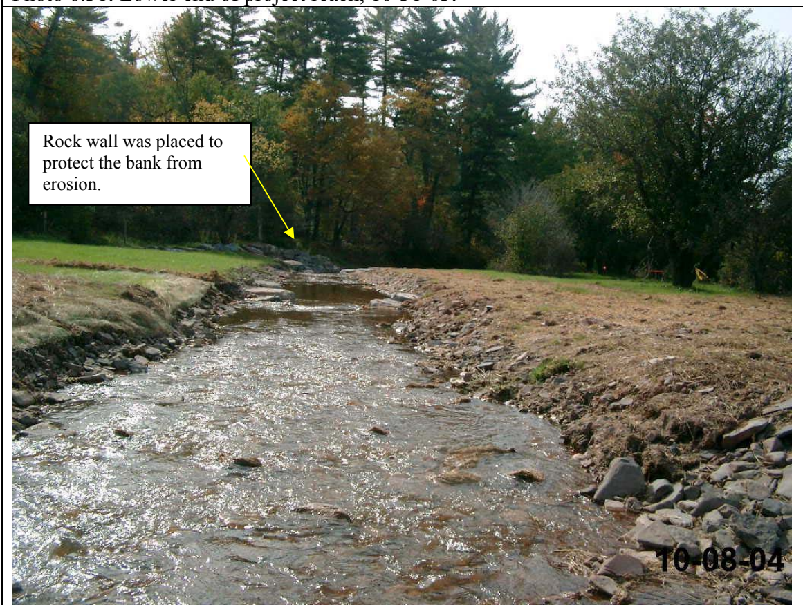
Photo 6.32: Looking U.S. at the end of the project, 10-08-04.
