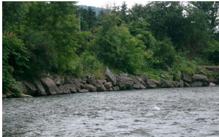
Figure 4.2 Example of streambank riprap above County Route 2 bridge in Delancey
