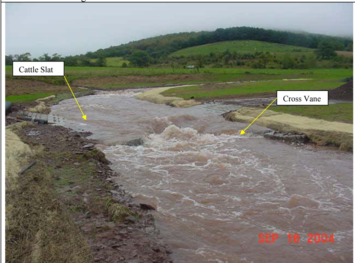
Photo 6.36: Looking U.S. at cross vane and cattle slat, 9-18-04.
