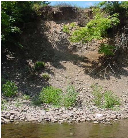
Figure 7.3.10 High eroding bank located approximately 3,300 feet upstream from private bridge.
