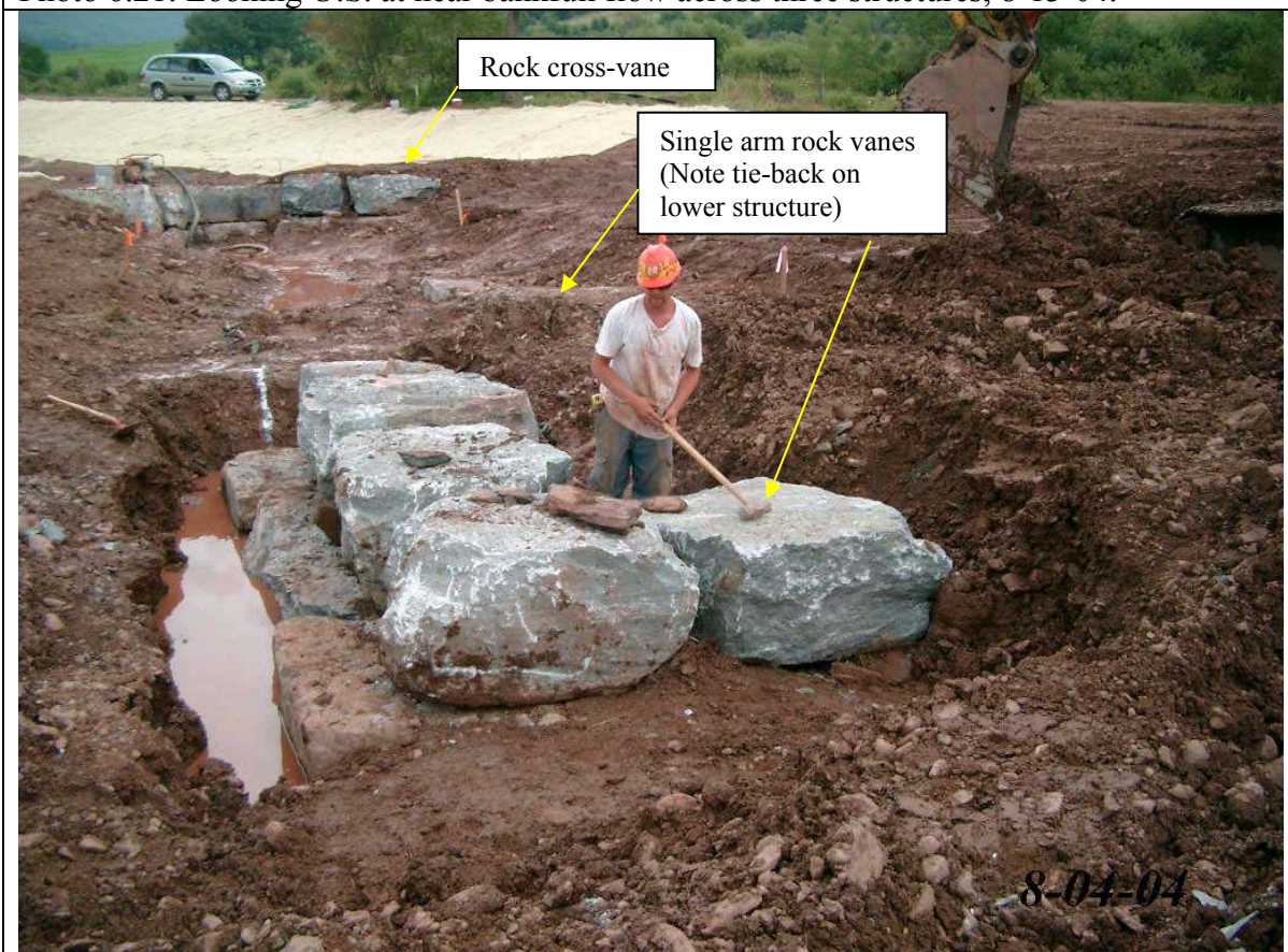
Photo 6.22: Looking U.S. the same three structures in photo 7 during construction, 8-04-04.
