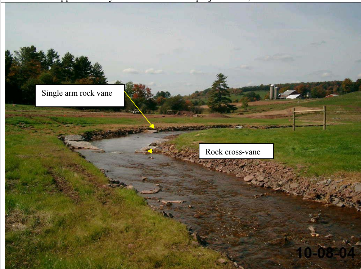
Photo 6.28: Looking D.S. at cross-vane approximate area as the above picture, 10-08-04.
