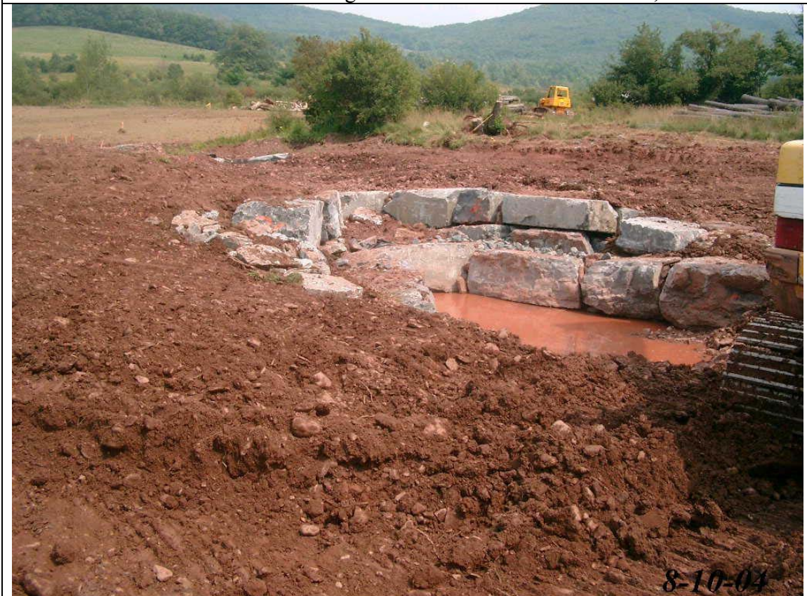
Photo 6.26: The double cross-vane structure during construction, 8-10-04.
