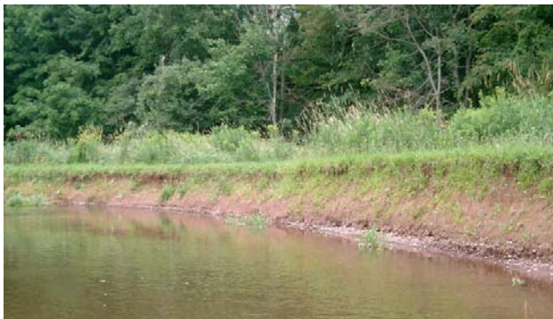
Figure 7.4.13 Poorly vegetated eroding bank located upstream from Peaks Brook confluence.
