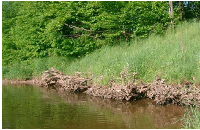
Figure 7.6.2 Root wad revetment that is located near the Delaware County Solid Waste Management Center.
