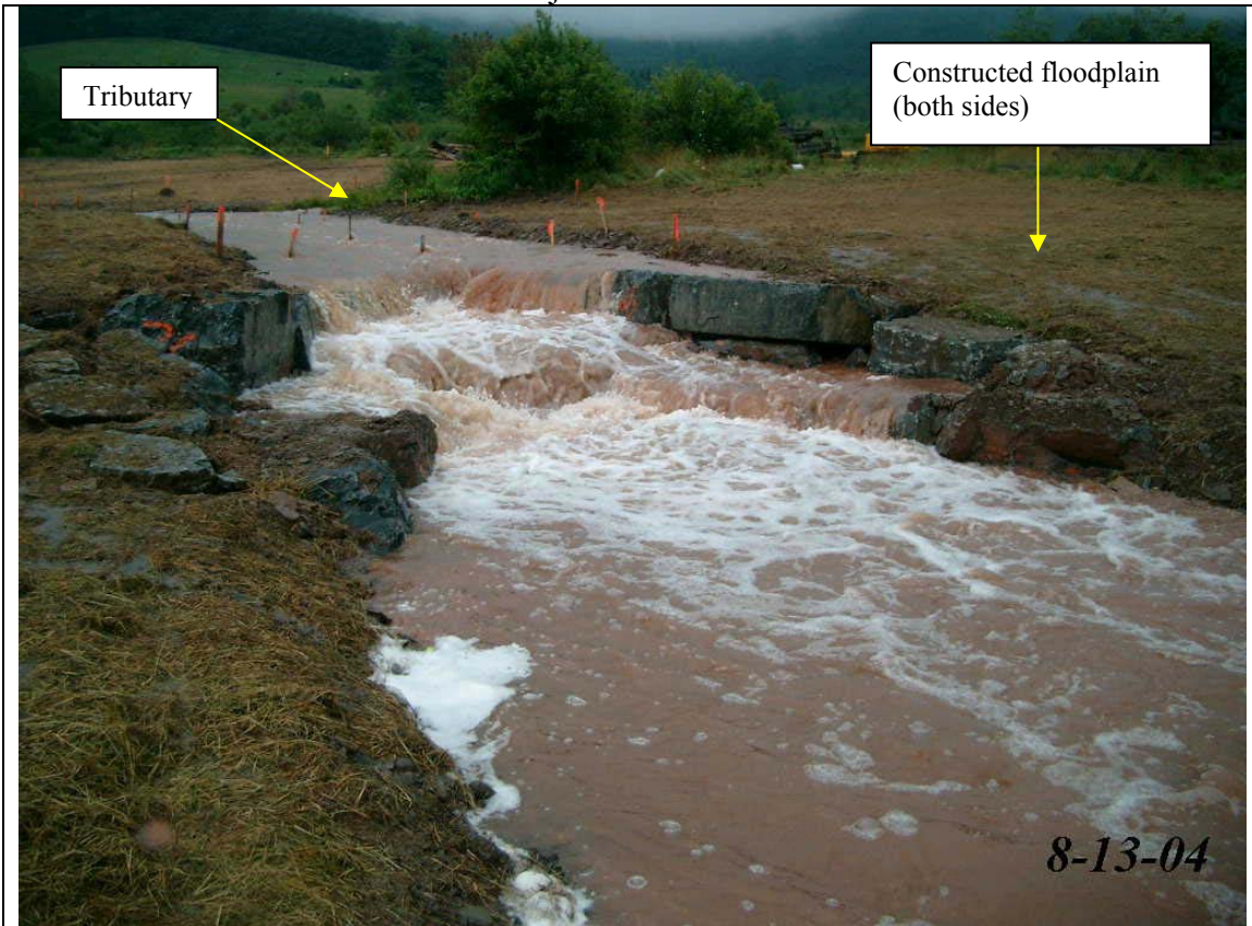
Photo 6.25: Near bankfull flow through the double cross-vane structure, 8-13-04.
