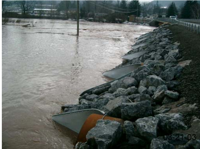
Figure 6.13 Floodplain relief culverts installed at County Bridge 2-1 in Delancey. Photo taken looking upstream, March 21, 2003
