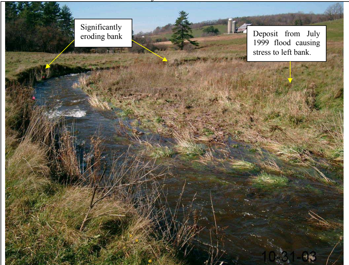
Photo 6.27: Approximately at the middle of the project reach, 10-31-03.
