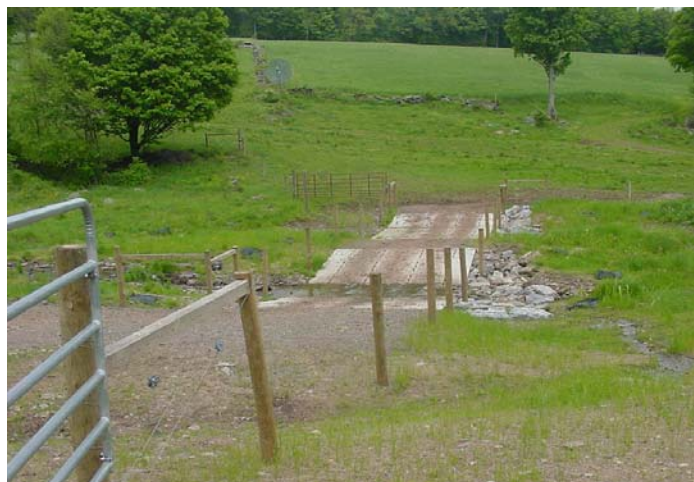
Figure 6.10 Fenced livestock crossing with animal walkway.
