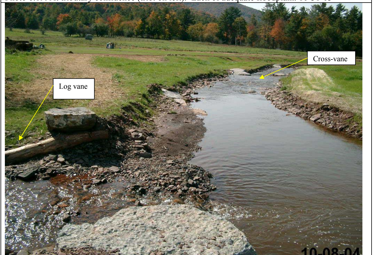
Photo 6.20: Tributary on the left with log vane enters town brook at cross-vane.
