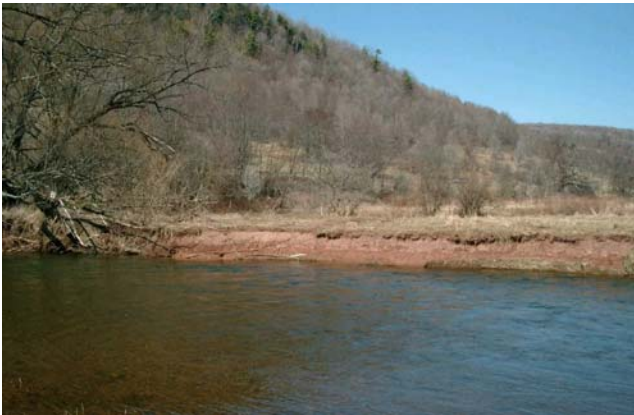
Figure 7.3. 15 An eroding bank downstream of railroad bridge where bank pin #34.3 is located.
