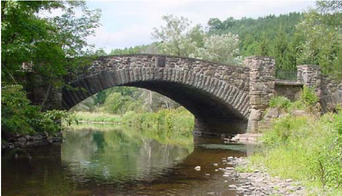
Figure 7.3.12 Looking downstream at County Bridge 18-6.
