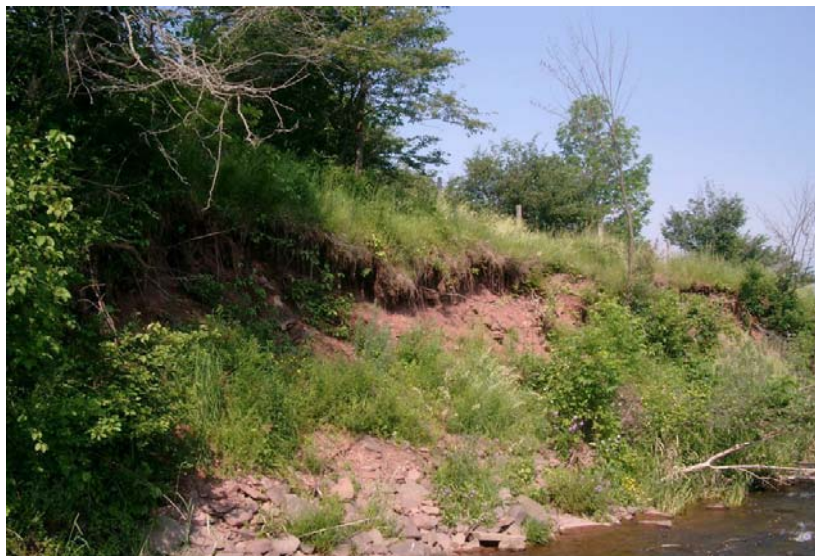
Figure 6.15 High eroding bank on Town Brook just below cross-section 10.
