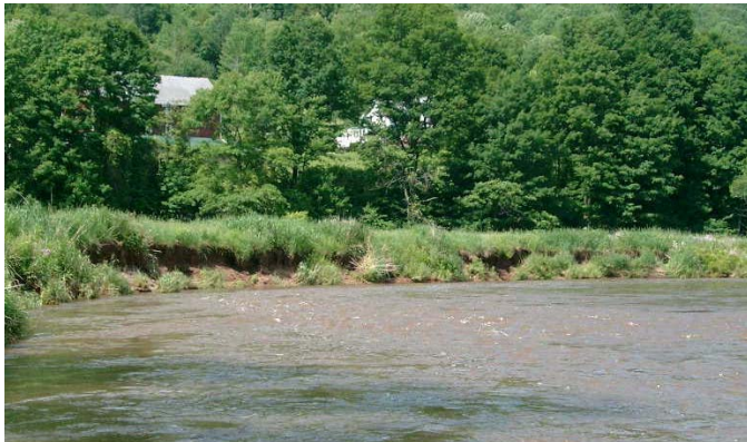
Figure 7.6.5 Poorly vegetated left eroding bank located approximately 1,500 feet upstream from Marvin Hollow confluence.
