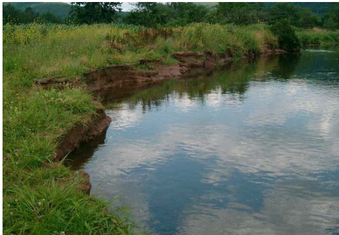
Figure 7.5.3 Eroding bank upstream from Bagley Brook confluence.
