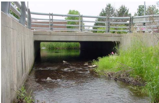
Figure 7.2.4 Looking downstream at NYS Route 23 Bridge.
