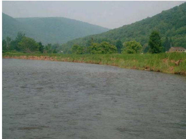
Figure 7.6.3 Poorly vegetated right bank that is eroding located approximately 1,500 feet downstream from Bonnefond Road.
